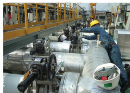
Loading arm construction
